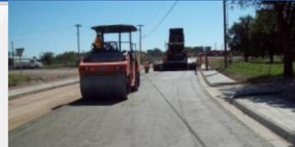
Grape Creek Road – San Angelo, TX
